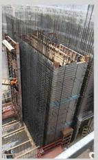
Reinforcement, normally steel, is placed in concrete to provide the tension strength of the finished component.
