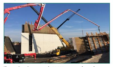
The project incorporated 90,000 square feet of custom engineered form work for walls with complex geometries and heights varying from 3 meters to 20 meters high.
