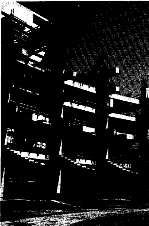
◀ Cantilevered beams provided unobstructed views.
