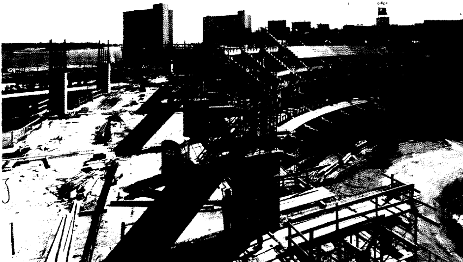
◀ 48 cast-in-place main frames form the basic structure.
