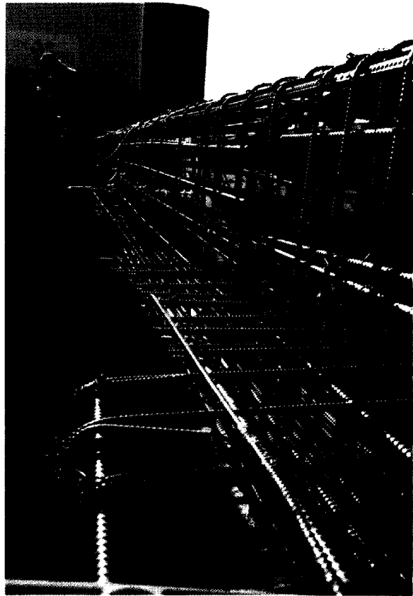
Epoxy coated rebar was used in areas vulnerable to corrosive salts.
