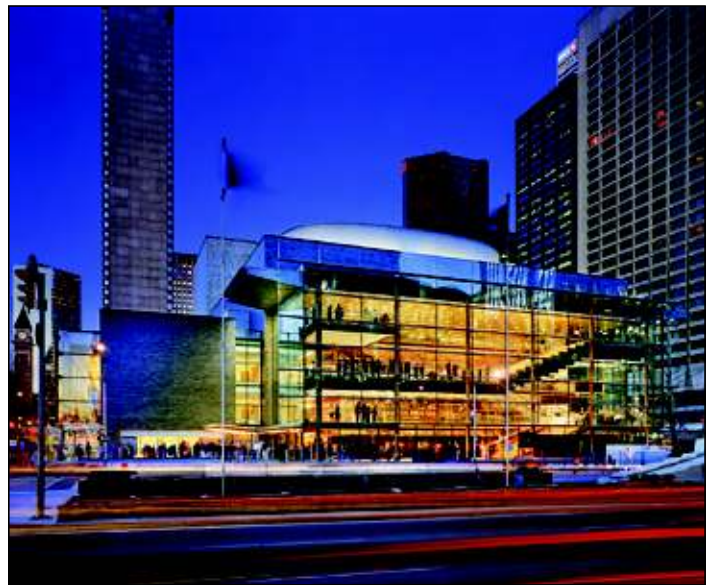
2006 Ontario Concrete Award winning project for Structural Design Innovation
