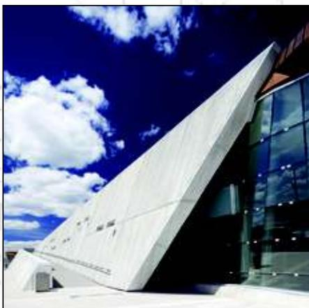
To create the Vertical Board Pattern, rough sawn boards of random widths, lengths and thicknesses spaced with varying gaps insured that the concrete would ooze out between boards. With the Random Plywood Pattern, the contractors were instructed to find old and discarded plywood from previously used formwork,
